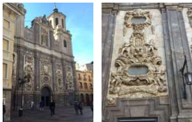
Fig. 2. The Santa Isabel Church and sculptures fragment at the façade (right)
